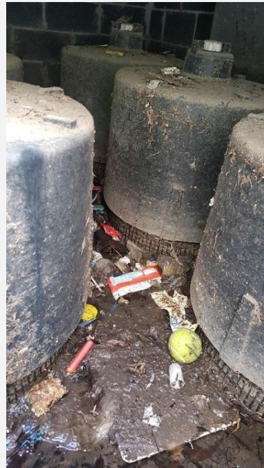
Figure 2: Examples of gross pollutant interception within OP StormFilter chambers in Australia including leaf litter in image (a) and other gross pollutants including litter in images (b) and (c)
