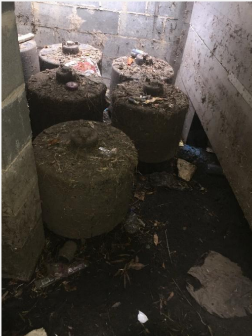
Figure 2: Examples of gross pollutant interception within OP StormFilter chambers in Australia including leaf litter in image (a) and other gross pollutants including litter in images (b) and (c)
